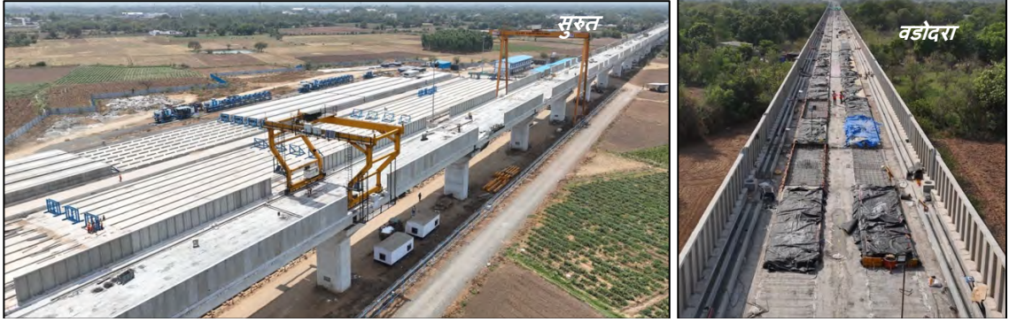
Noise Barrier Installation Work in Progress, Gujarat
